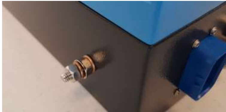
Figure 2 - Equipotential bonding point location
