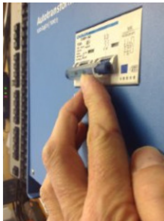
Switch the MCB ON
