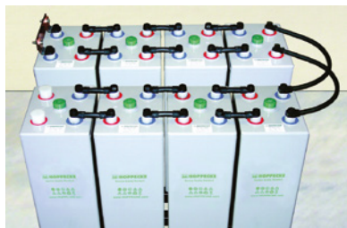
Fig. 5-15: Using row connectors and step connectors
