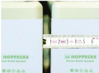
Fig. 5-14: 10 mm clearance between the batteries
